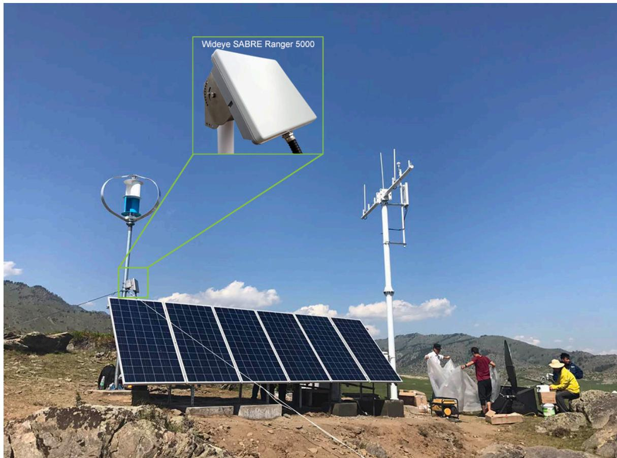
A photo showing the setup using Addvalue Wideye SABRE Ranger 5000 BGAN terminal to implement the Kanas Tourism Securities Monitoring Platform System.
